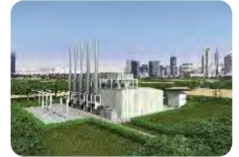
Large CHP power plants
