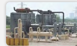
Gas Compression (low emissions) Barnett Shale, Dallas/ Fort Worth, TX 2700 hp | 2 x L5794GSI
