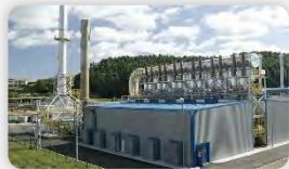
Steel Furnace Gas Arcelor Mittal | Avilés, Spain 20.4 MW | 12 x J620
