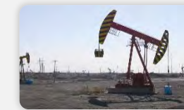
Remote Power Jidong oilfield, China 4000 hp | 3x L5794GSI
