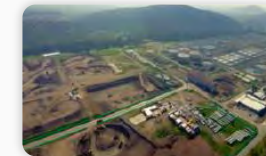
Sewage gas Santiago Basin, Chile 7.3 MW | 3x J620
