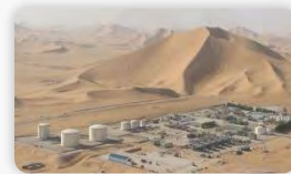
Gas injection Algeria F3524GSI
