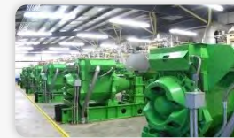
Landfill Gas Ox Mountain (CA, USA) 11.5 MW | 6 x J616
