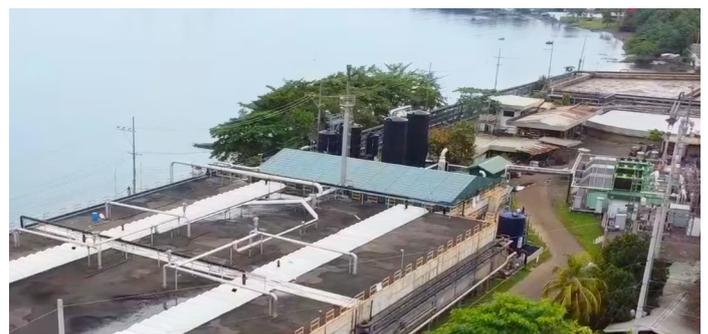
Today, manufacturing wastewater from the pineapple processing is converted to biogas for the facility's new CHP plant. Installed in 2015, two Jenbacher J420 engines running on biogas provide 1,411 kW of electricity and 1,594 kW of thermal energy that preheats the boiler feedwater. Biogas also powers a Jenbacher J320 that was added in 2019 to provide an additional 1,059 kW of electricity.
